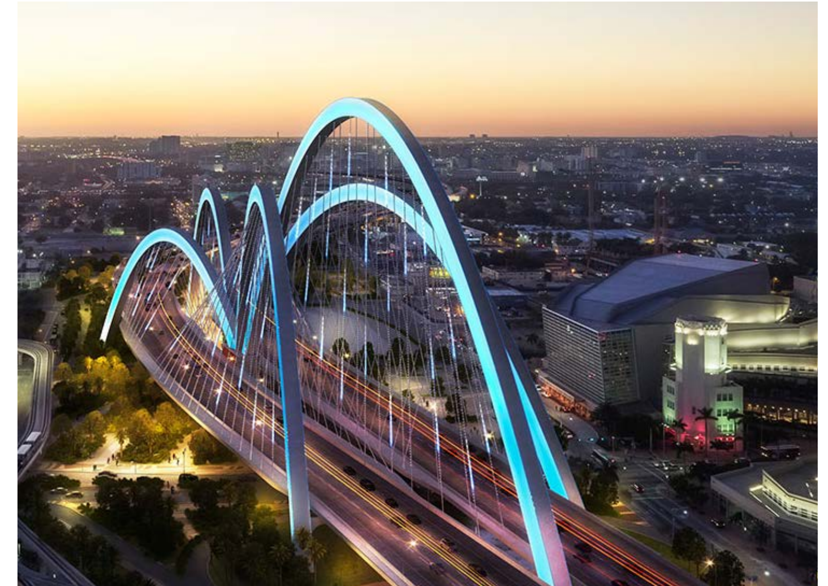
I-395 SIGNATURE BRIDGE
